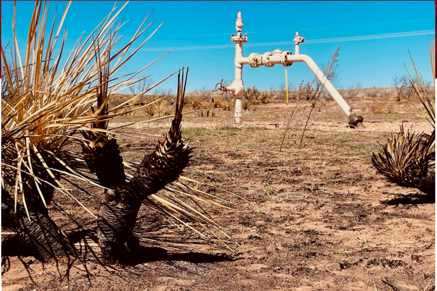
Cleared well site in Moore County
