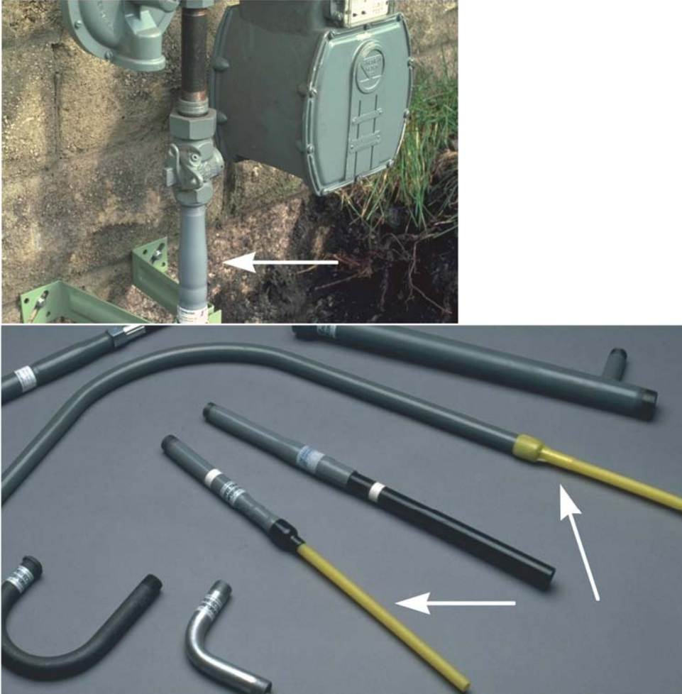
Figure VI-17: Anodeless risers
