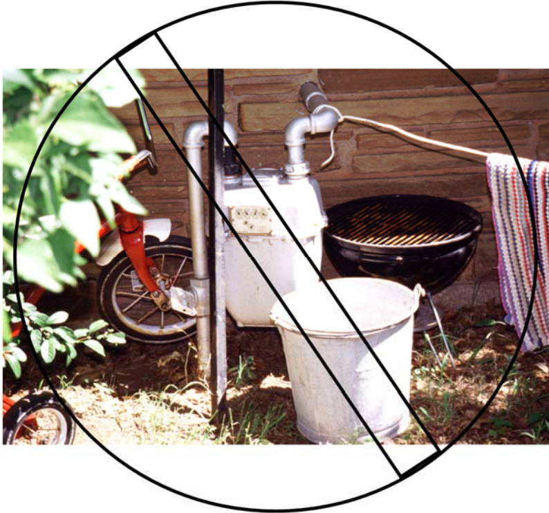
Figure III-17 Shorted Meter Set.
