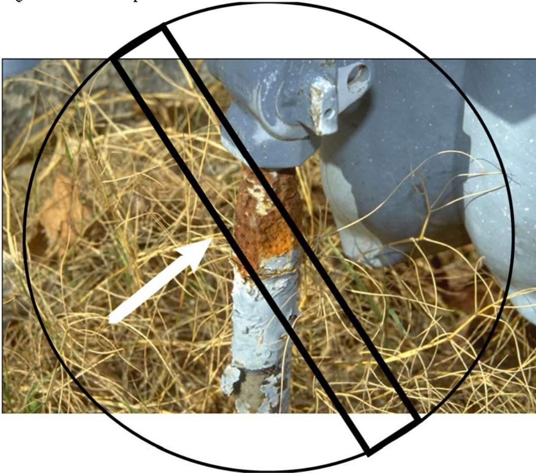
Figure III-24 Atmospheric Corrosion
